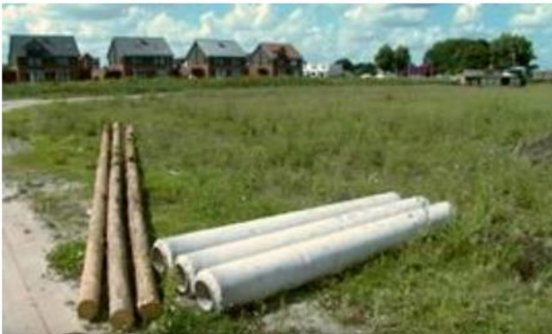
Timber piles and concrete extension piles
