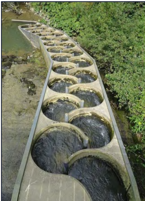
Fish ladder ensures natural movement for fish Figure 4: Example Fishladder [2]
