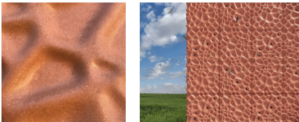
3D biocomposite facade for Amsterdam Pavilion
