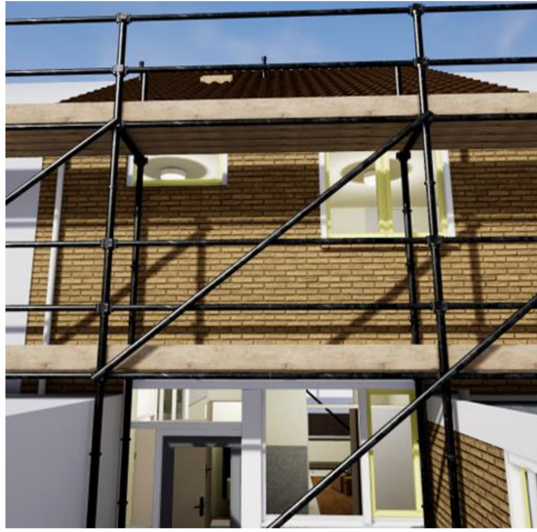
Scaffolded home during renovation
